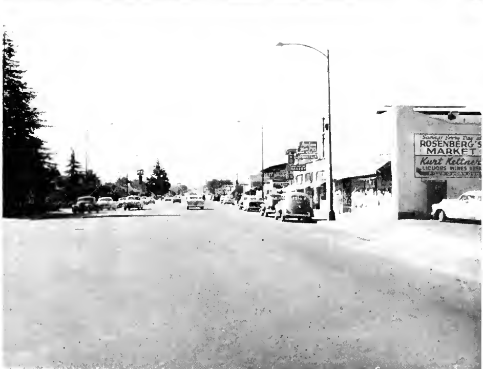
UPPER—Lincoln Avenue between Brace and Minnesota, looking south, before improvement. LOWER—Same location after improvement.
